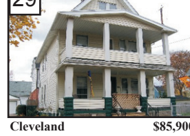
29 Cleveland $85,900 POSITIVE CASH FLOW! Investment Opportunity! Double with vinyl siding is ready for you! Fenced yard. Awnings. Owner occupied.
