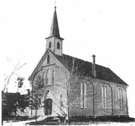
Sacred Heart of Mary Church, which was destroyed by fire in 1907.
