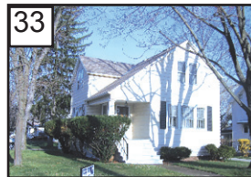
33 Cleveland $109,900 CLASSIC COLONIAL! Rehabbed Colonial with many updates. 4 bdms, 1-1/2 baths. New win., furnace & C/A, elec, copper plumbing, paint & carpet. Remodeled kitchen, bath. Eric Ebsch 216-376-3067
