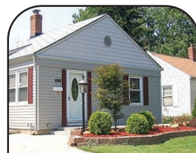
Cleveland $99,900 Spectacular Upgrades & Decor LAID OUT FAMILY ROOM
