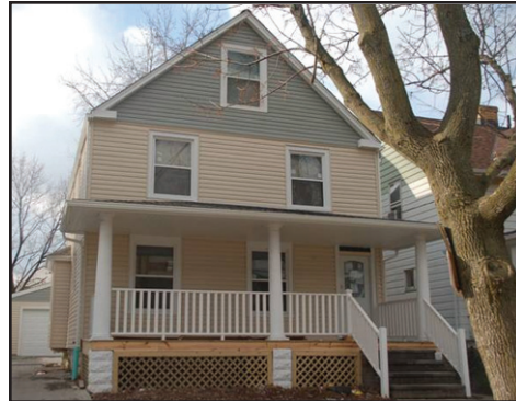
OBCDC-renovated home, 3307 Altoona Ave.
