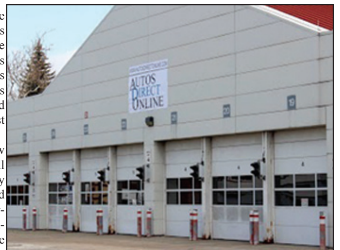
Since February, Autos Direct Online cars, rather than GCRTA buses, have been housed in this huge garage at 4371 Pearl Rd.
